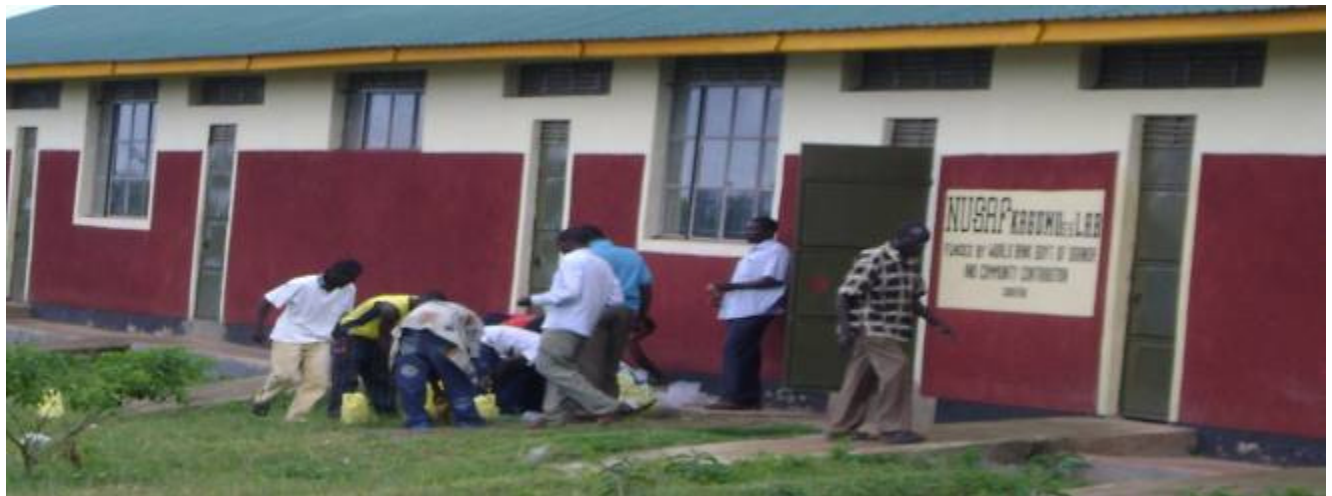
Kagumu secondary school completed laboratory is in use.
